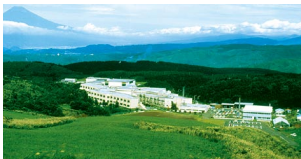
The Nakaizu Rehabilitation Center
